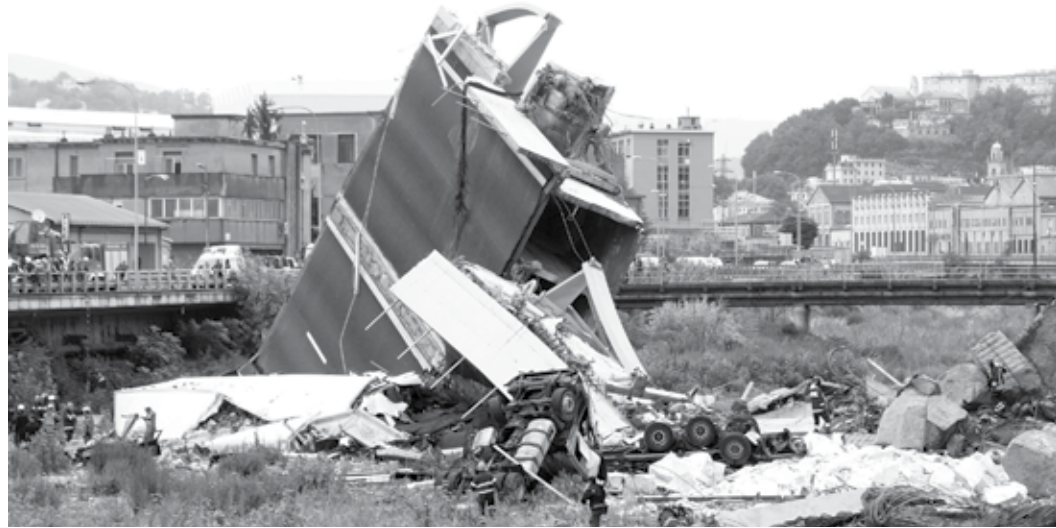
Rescuers are at work amid the rubble of a section of a giant motorway bridge that collapsed earlier
